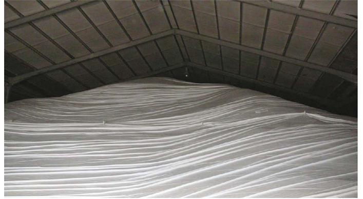
Insulation of roof and correct sheeting prevents condensation and water uptake.
