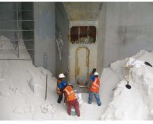
Removing damaged product from cargo hold
