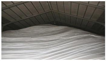
Insulation of roof and correct sheeting prevents condensation and water uptake.
